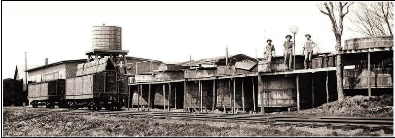
A typical salting station consisted of a fenced off area, 10 to 30 giant wooden brining tanks with a raised walkway around them, a pump house and water tower for a ready supply of fresh water, and a storage building to hold tools, office space, and a huge amount of salt. This Heinz salting station in Wisconsin was typical of the ten similar plants along the NKP. Marquette County Historical Museum collection.
