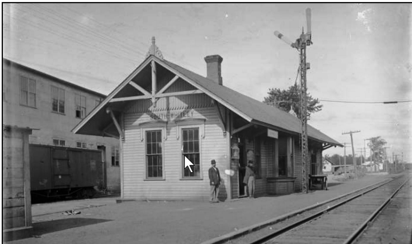
#9. The Nickel Plate depot in South Whitley was a completely common "Class Three" combination depot, built around 1884 and found all over the NKP mainline.
