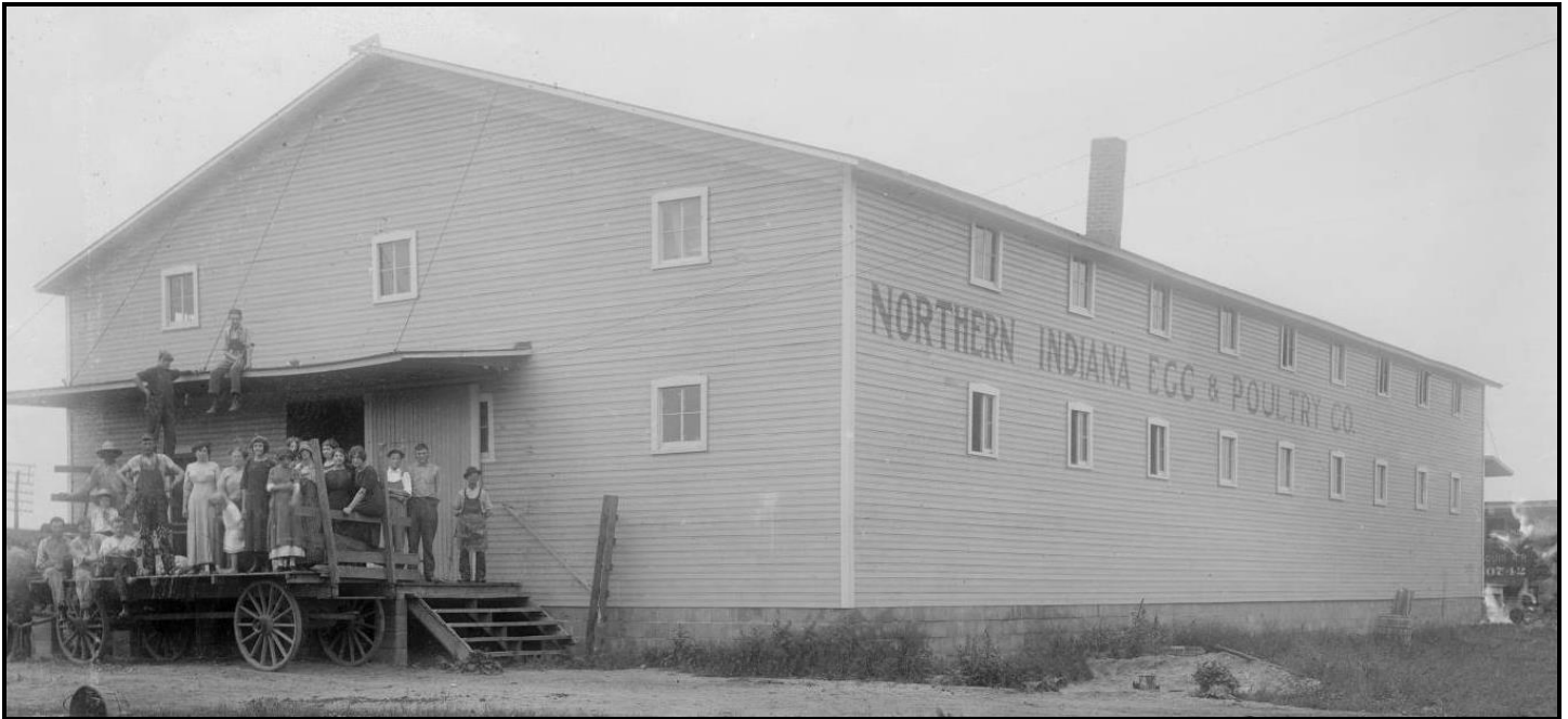
#2. Next to the stockyards was the Northern Indiana Egg & Poultry Co. Mainly dealing in fresh eggs for the Chicago market, the company also sold dressed and frozen chickens. This photo shows the “street side” of the building; at the far right distance is a NKP boxcar waiting to be loaded with crates of eggs.
