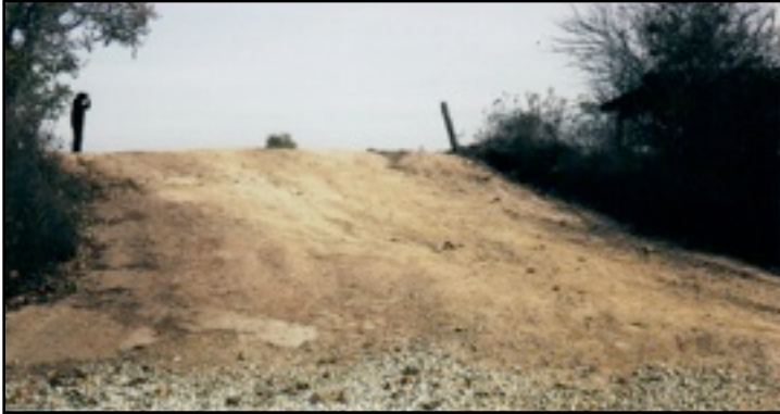
Fig. 9 - View looking up the ramp to where the loads are transferred. Note the pole to the right of center was probably used as a backing aid.
