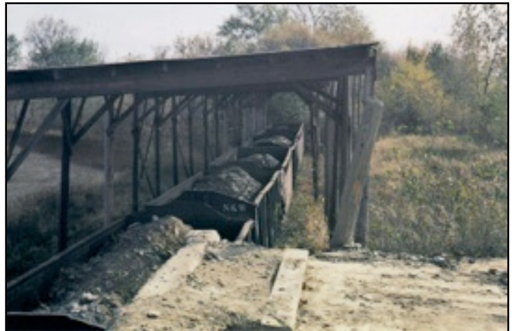
Fig. 12 - Another 1988 view of the shelter. Here along the south row of poles can be seen the apparent inset of the further poles by about three feet or so. This leads me to wonder if this shelter may have been built in two sections as the need grew for more clay. Also visible here is the sighting pole and one of the tire stops.
