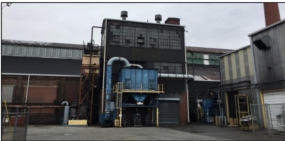
Photo of the Coke Conditioning Building as it exists today.
