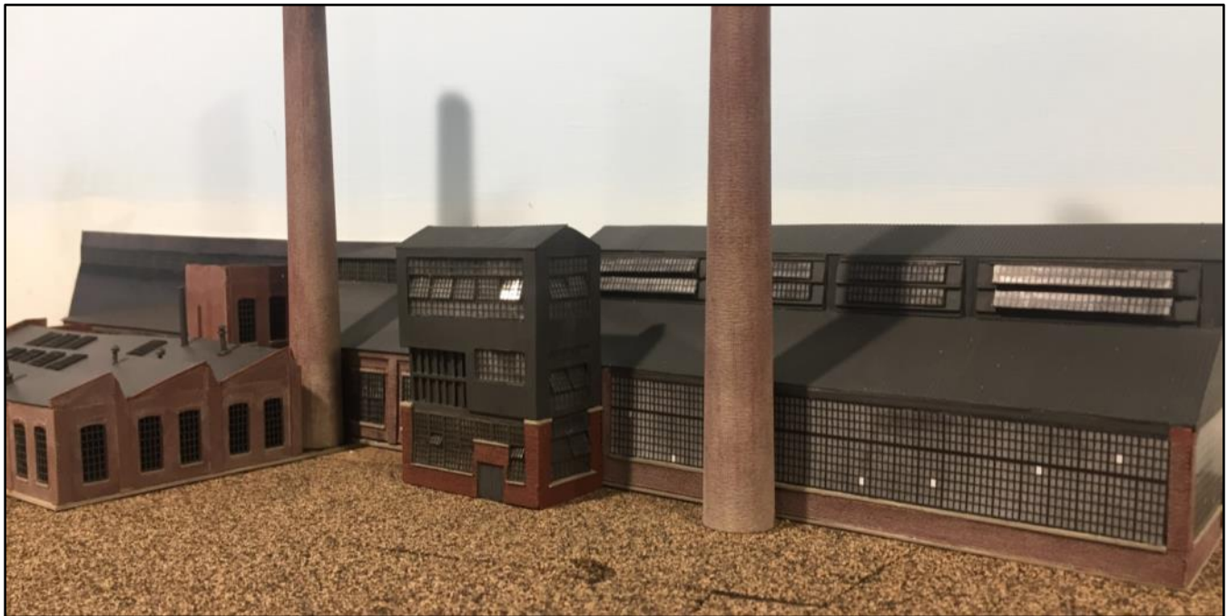
The completed CCB on the layout.
