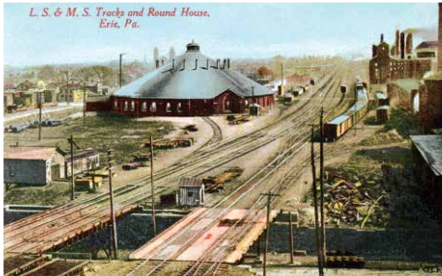
The Lake Shore & Michigan Southern was destined to become the principal railroad through Erie, which it remains today under CSX auspices. A colorized postcard view looking eastward shows a fully enclosed, 360-degree roundhouse facility. The view appears to be from a vantage point near State Street; the French Street underpass is in the foreground. JERRY D' AURORA COLLECTION
