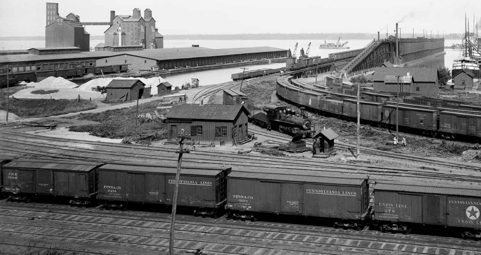
ABOVE: Dock facilities at Erie were dominated by the mighty Pennsylvania Railroad interests, as is evident in this scene from early in the 20th Century. The Anchor Line boat docks are at upper left, but everything else is PRR in this photo. Prominent is a coal-unloading facility in which loaded hoppers were hoisted by cables up an incline track—with safety backstops much like the chain-lift storage of a roller coaster’s first hill—and onto the dump tracks for transfer of coal to lake boats. At right, ore is being transferred from lake boats to temporary storage piles for later transfer to hoppers or gons destined for steel mills in Pittsburgh. FACING PAGE, TOP: A closer look at the same docks reveals “whirleys” unloading ore from lake boats and into gons or the storage piles. The whirley nickname stems from the ability of the steam-powered cranes to rotate on spot to transfer ore from boat to gons or piles. BOTH PHOTOS, JERRY SKRYPZAK COLLECTION
