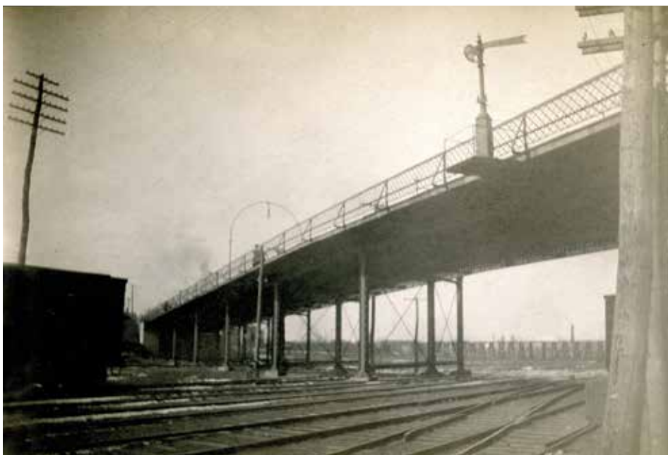
LEFT: A 1909 photo looking north into PRR's Warfel Yard shows, in the distance, the only known photo of the NKP's wooden trestle across the yard. The trestle was replaced by a combination of fill work and girder bridges as shown on the opening spread of this feature. Note how the semaphore signal has been mounted onto the roadway bridge. JERRY D' AURORA COLLECTION
