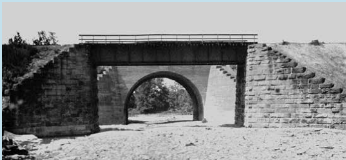
BELOW: Bridge 49 over Sixteen Mile Creek near North East, Pa., in 1918. The NYC's older, stone-block arch bridge is beyond. NATIONAL ARCHIVES
