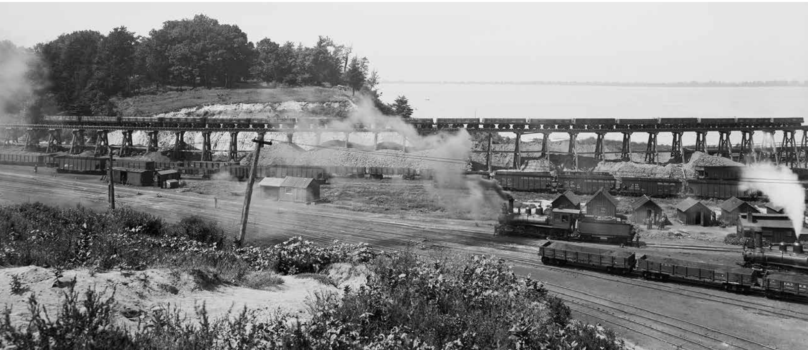
BELOW: The Erie & Pittsburgh (Pennsylvania Railroad) docks at Erie are shown in 1904. E&P 2-8-0s stand by for their next tasks. The E&P docks were the farthest west of the railroad docks at Erie. Note the three-truck gons on the trestle. JERRY SKRYPZAK COLLECTION
